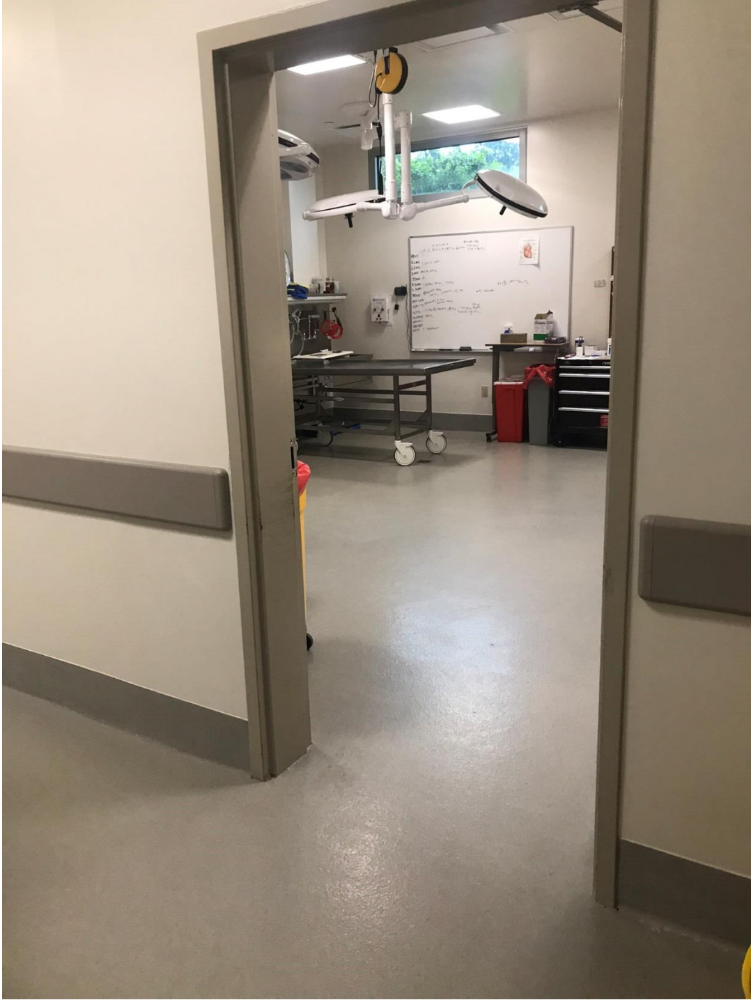
Area C Existing Door - Picture from Corridor
